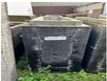
#502 • Concrete Water Tank Basin
