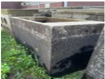
#501 • Concrete Water Tank Basin
