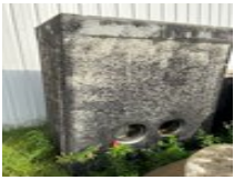
#500 • Concrete Water Tank Basin
