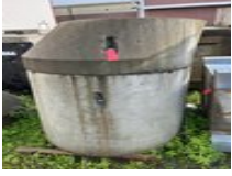
#497 • Concrete Water Tank Basin
