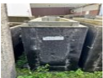
#504 • Concrete Water Tank Basin
