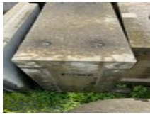
#505 • Concrete Water Tank Basin
