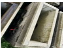
#503 • Concrete Water Tank Basin
