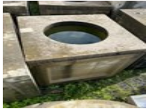
#506 • Concrete Water Tank Basin
